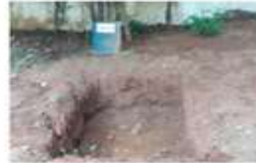
Rain Water Storage & Compost Pit
